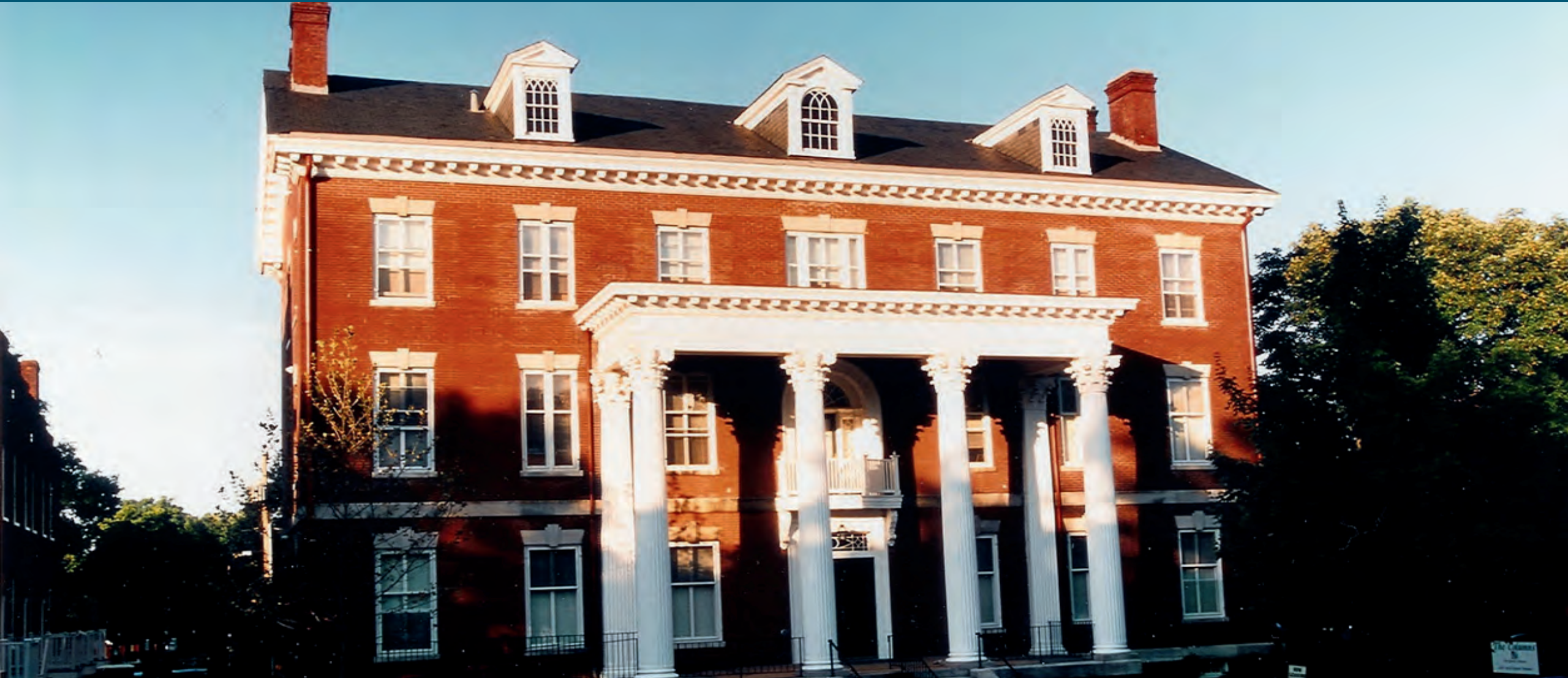
Columns on Grove Senior Apartments | Richmond, VA
