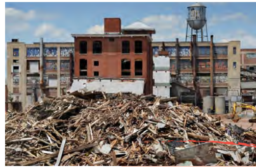
demolition of mill buildings
