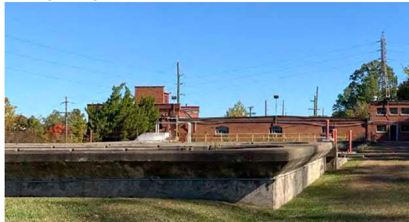
Sediment Basins looking east
